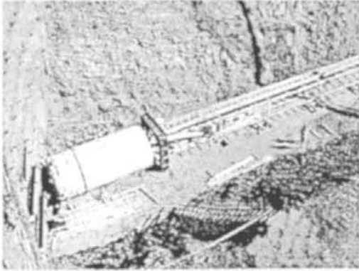
Figure 18. TBM at the Portal
