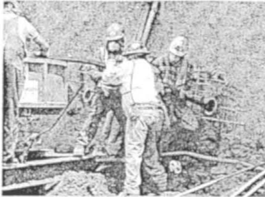
Figure 8. Installing Tieback
