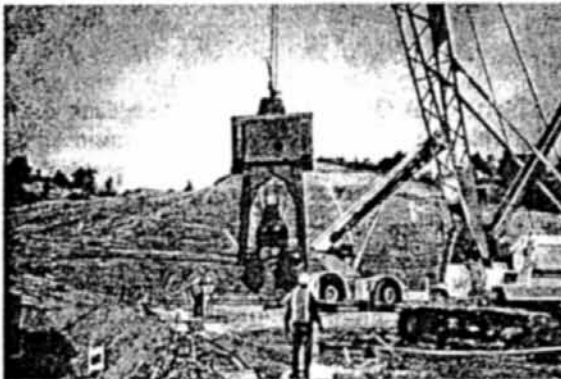
Figure 2. Excavation Using Clam
