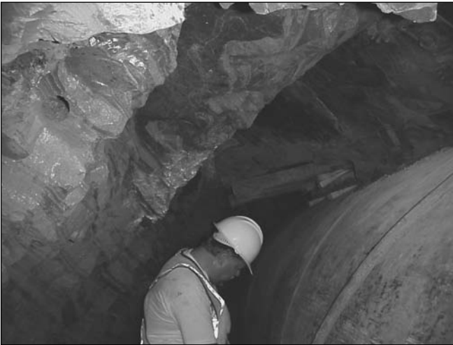
Figure 20. Hand mined cavern outside of TBM
