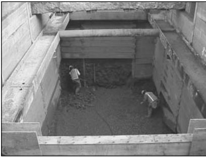
Figure 14. Tunnel access shaft
