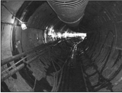
Figure 9. Segment lined tunnel
