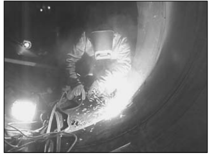
Figure 12. Welding steel pipe joint
