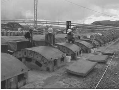
Figure 5. Segment casting yard
