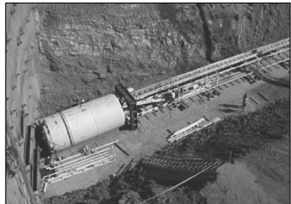
Figure 4. EPBM assembly
