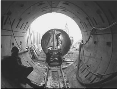
Figure 11. Loaded pipe carrier
