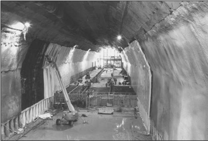
Figure 18. Construction of final invert and interior arch
