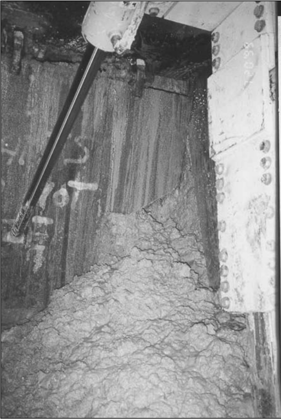
Figure 10. Flowing ground conditions in drift 4E
