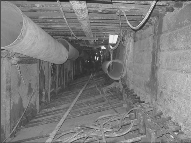
Figure 14. Threadbar reinforcement in drift 7W
