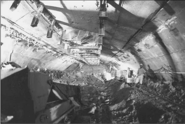
Figure 15. Excavation of first lift
