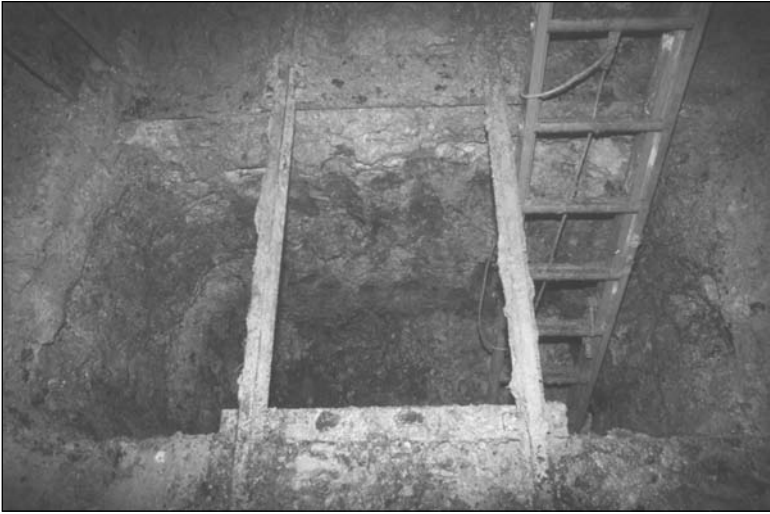
Figure 12. Foundation pier pit in drift 1E
