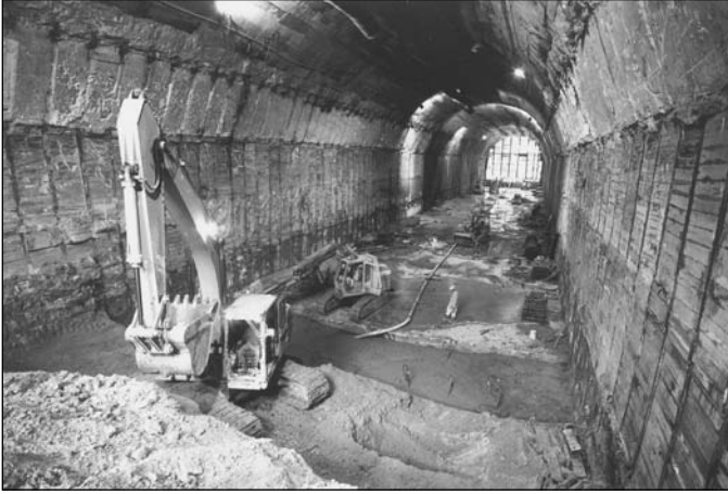
Figure 17. Excavation of lower lift
