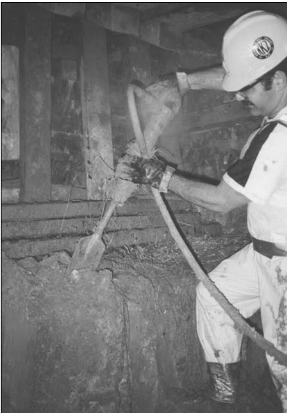
Figure 7. Hand excavation in drift G
