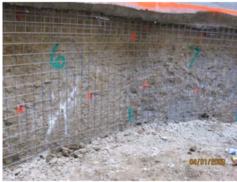
Figure 11. Wire mesh reinforcing for shotcrete
