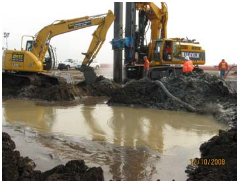
Figure 8. Fluidized slurry management at the receiving shaft.
