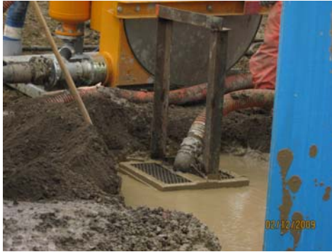
Figure 9. Fluidized slurry management at the jacking shaft
