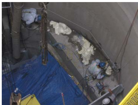
Figure 14. Hydrophobic grout injection in progress
