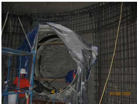
Figure 12. Structural reinforcing around the tunnel eye
