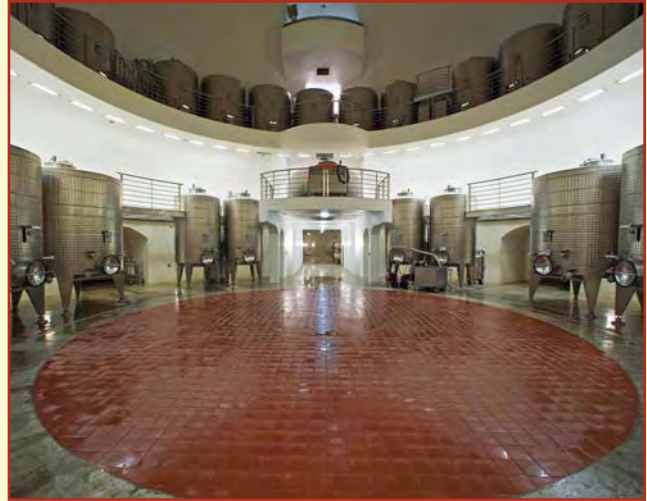
The fermentation dome is the world's largest underground reinforced structure at 72-ft diameter and 54-ft high.
