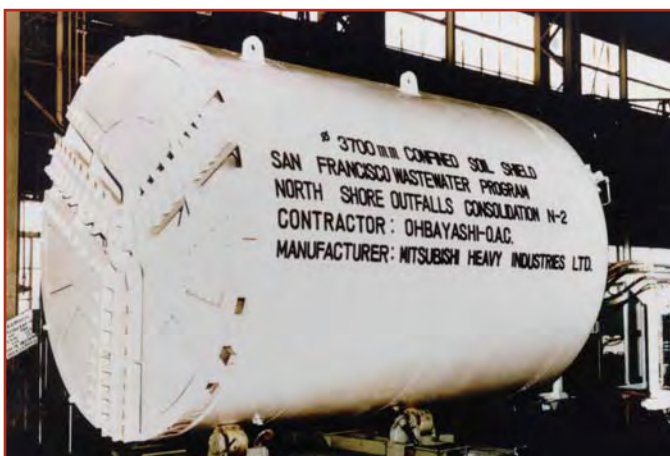
The N-2 Tunnel utilized the first Earth Pressure Balance TBM in the United States in 1980
