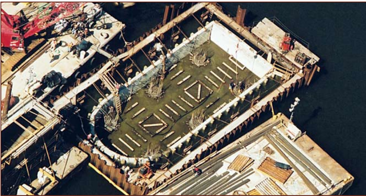
Figure 5: Precast Bathtub Nearly Complete. Courtesy of Morgan Kaolian/Aero, Inc.
