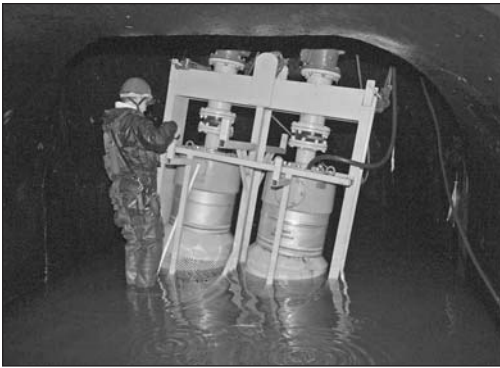
Figure 5. Dewatering pumps at the base of the working shaft
