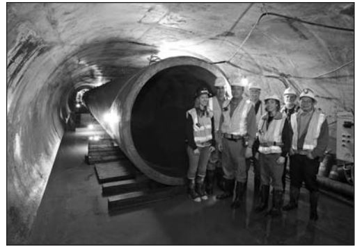
Figure 4. Combine ambient tunnel light with camera flash to create balanced underground photographs. In this image of East Bay Municipal District and Jacobs Associates personnel in the new Claremont Bypass Tunnel, the camera flash was bounced off the crown of the tunnel to light the subjects while reducing reflections off of the safety vests. (Photo used with permission of the East Bay Municipal Utility District.)
