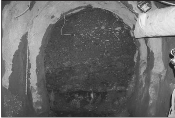
Figure 8. Mixed face condition
