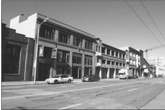
Figure 3. Existing buildings on Townsend Street above DTX alignment
