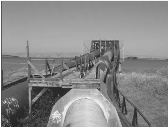
Figure 2. Bay Division Pipelines 1 and 2 at shoreline in East Palo Alto
