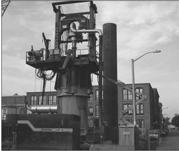
Figure 2. Wirth pile top rig
