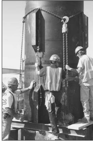
Figure 6. HDPE being installed as the inner member of composite liner
