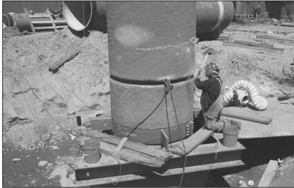
Figure 5. Welding 5-foot diameter concrete pipe liner installation—note clamps “hanging” pipe vertically
