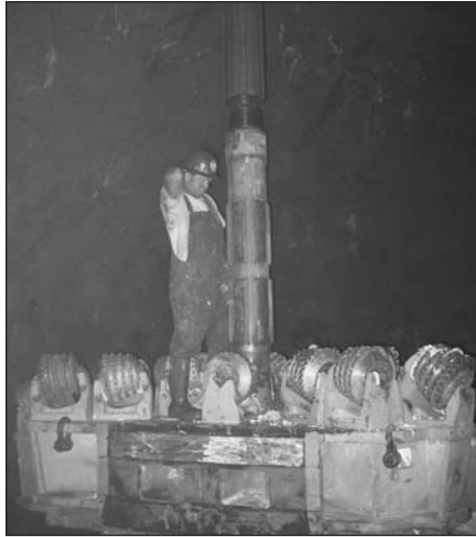
Figure 4. Raise bore reamer (144-inch) prior to commencing drop shaft excavation
