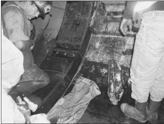
Figure 6. Installation of steel ring affixed with inflatable grout bags
