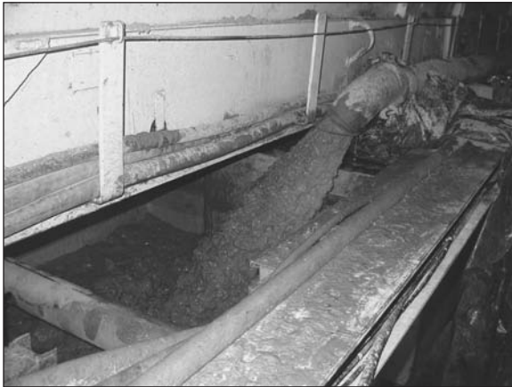
Figure 4. Excavated material discharged into muck cars
