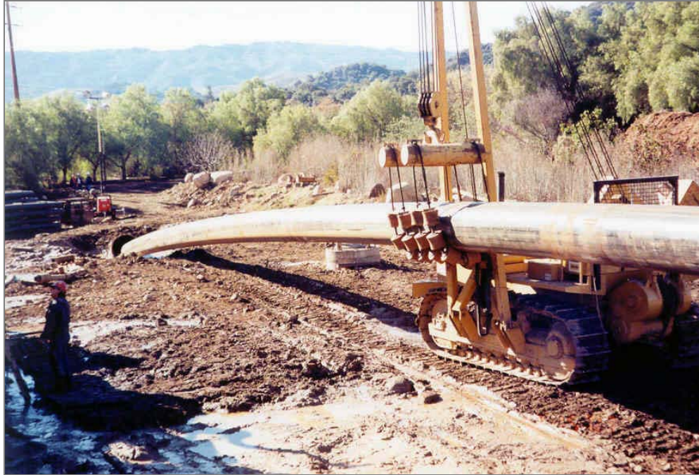
Casing Pull Back 30" – 3,200± feet 1 day
