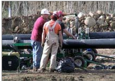
HDPE Carrier Pipe Assembly, Installation and Casing Grouting 2 weeks
