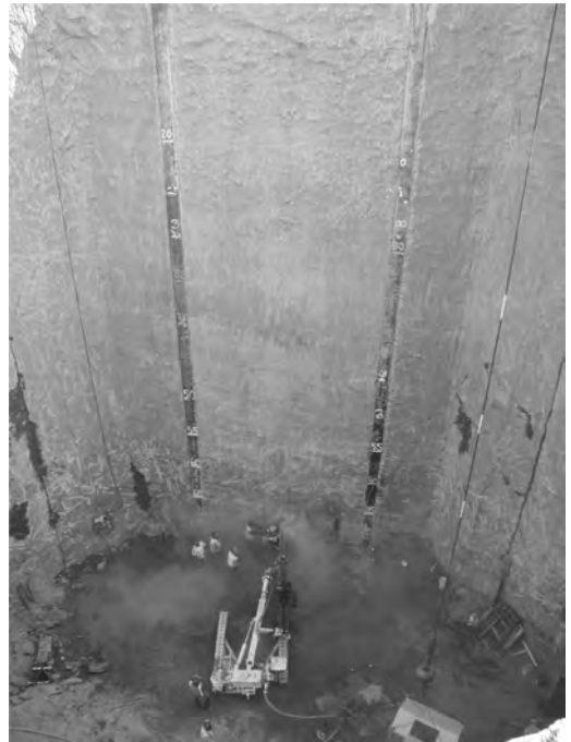
Figure 13. Drilling for rock anchor installation.
