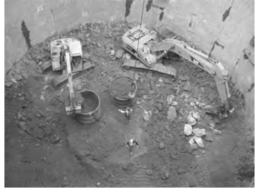
Figure 11. Excavation in rock.
