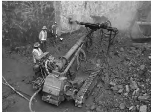
Figure 12. Drilling weep holes in the slurry wall.
