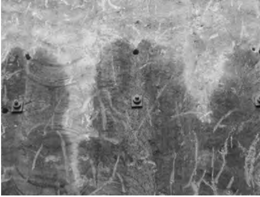
Figure 14. Weep holes drilled through the slurry wall.
