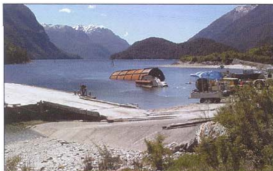
Delivery in Lake Manapouri of the steel tube mock-up of the tunnel section, which was used for trials of the bulkhead installation.
