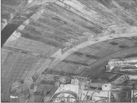
Figure 4. Installing Type C steel sets
