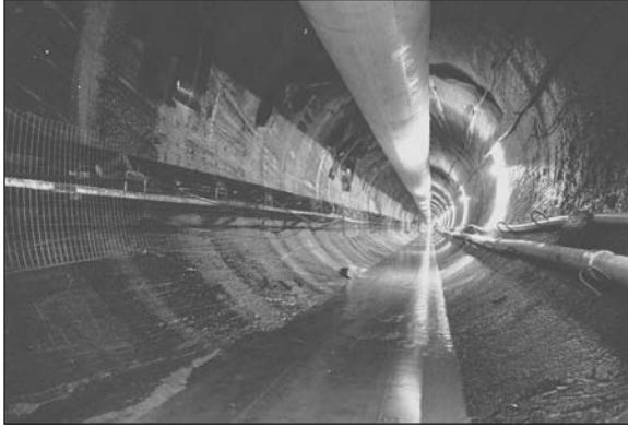
Figure 1. Chattahoochee hard rock tunnel
