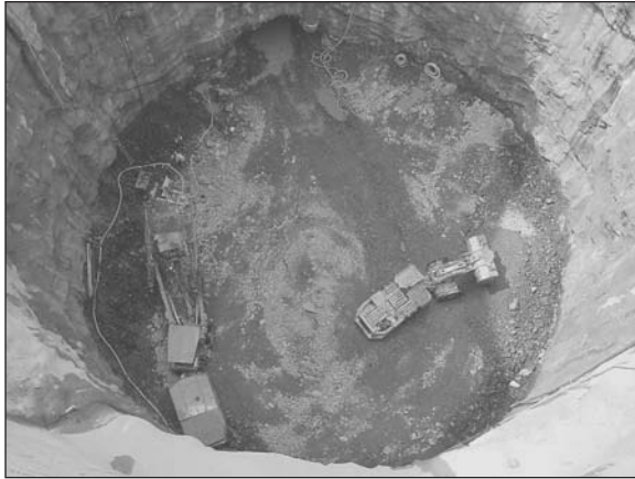
Figure 2. Pump station shaft during drill and blast tunnel excavation
