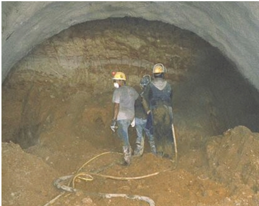
Shotcrete used successfully for initial support in a soft-ground tunnel
