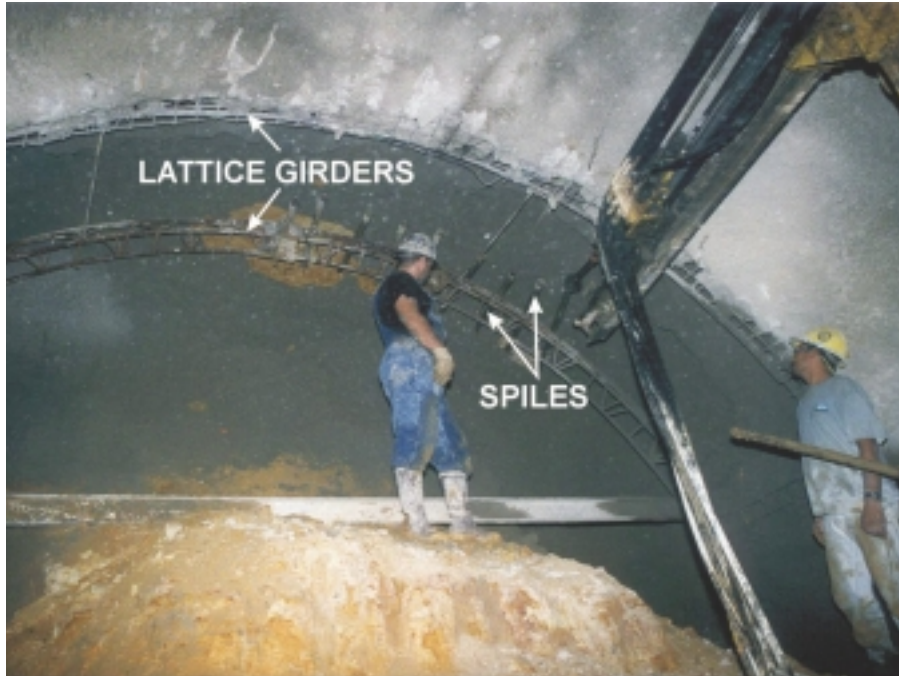
Short headings and spiles being used to control unstable ground
