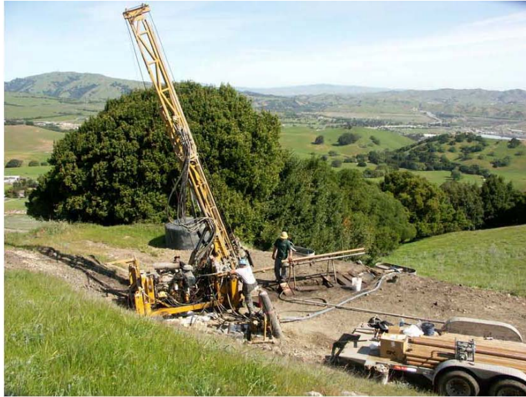
Figure 3. Drill Rig at Boring CB-8
