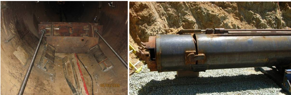
Figure 4. Examples of rods used for steering control. Dywidag bars inside the casing to make the casing stiffer (left). Pull rods used for steering control of auger bores (a similar concept can be included with microtunneling) (right).
