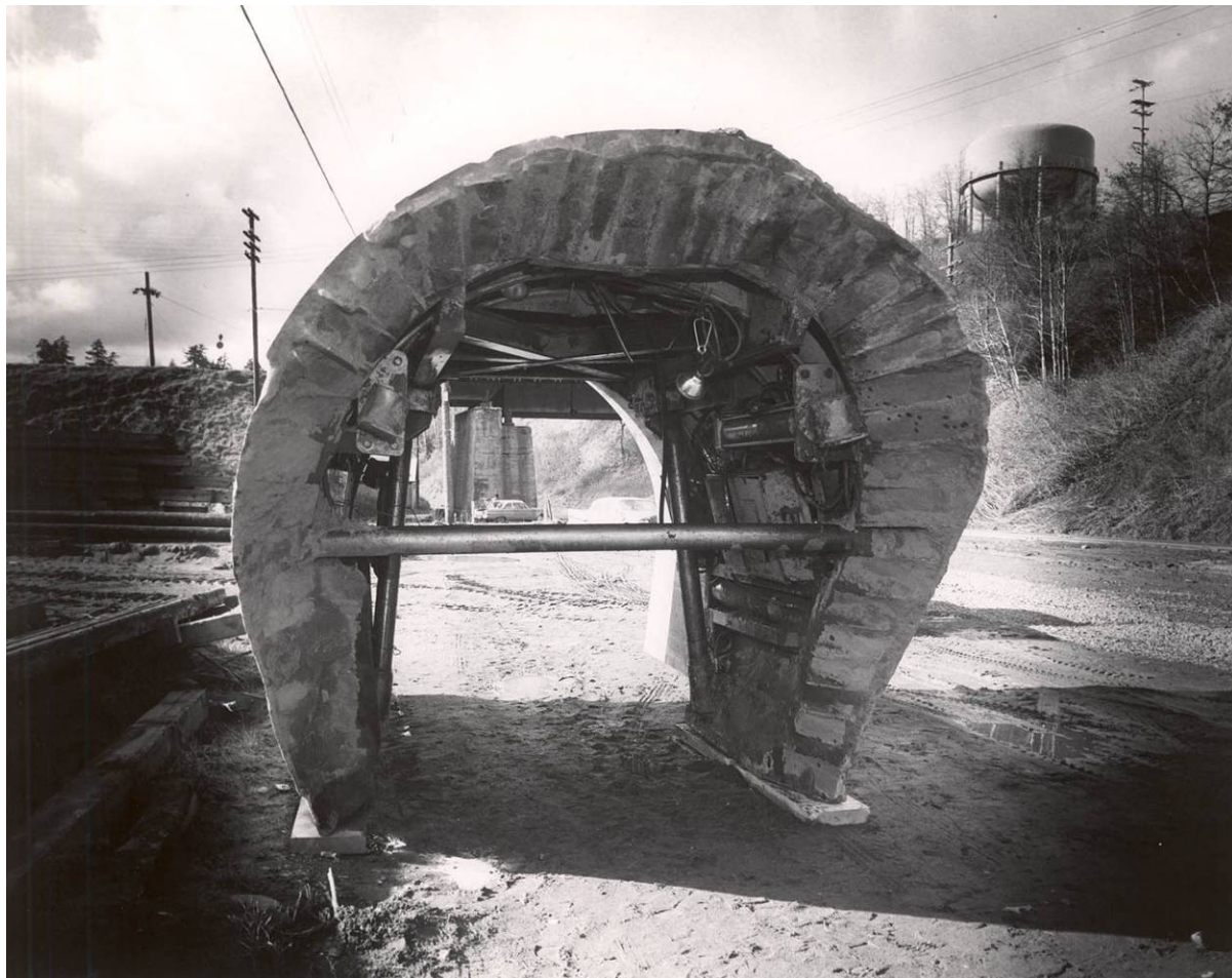
Figure 3. Front view of Portsmouth Tunnel open-face pneumatic shield with overhanging canopy (photo used with permission of the City of Portland Archives and Records)
