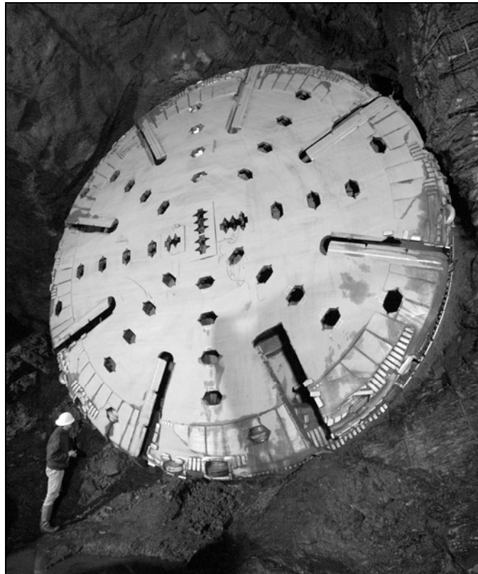
FIGURE 3. TBM cutterhead following hole-through at the Foundry shaft (photo by Sue Bednarz).
