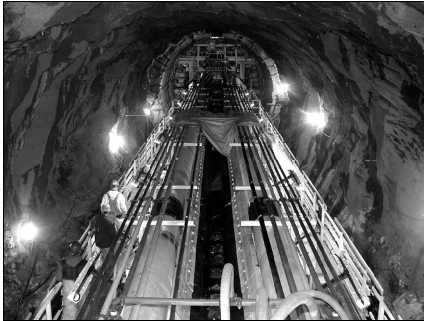
FIGURE 2. TBM in starter tunnel.
