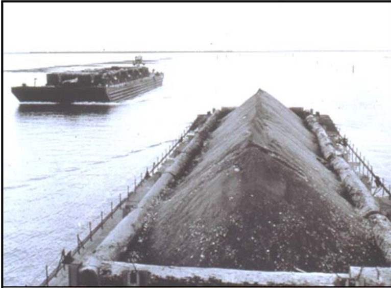
Figure 4- 1950's Causeway Construction
