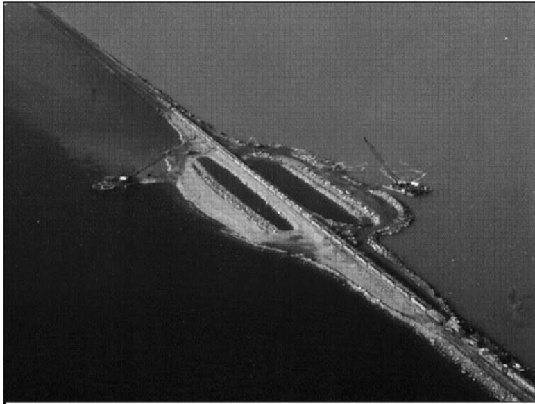
Fig 5: MP748 Final Berm Configuration
